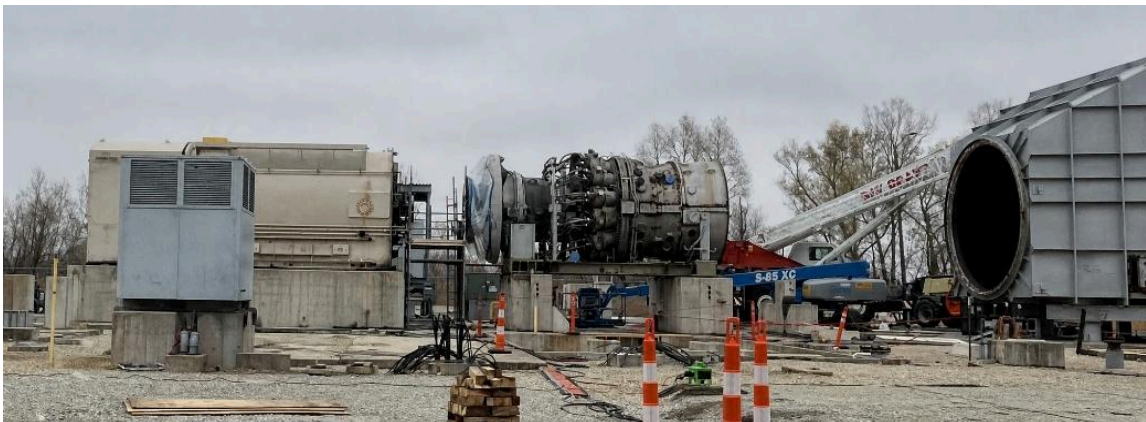
Figure 4: GE 7FA Gas Turbine After Dismantling
