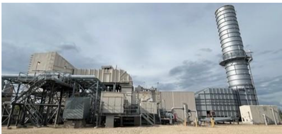
Figure 1: GE 7FA Gas Turbine Prior to Dismantling
