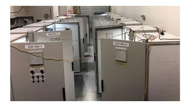
(CPwE) with Device Level Ring (DLR) architecture specified by Rockwell Automation. Each panel has two (2) 1783-ETAP1F embedded switches for the Device Level Ring (DLR) over fiber between the panels. The SCP master panel has two (2) Stratix 5700 managed Ethernet switches.1756-EN2TR modules are dedicated to the DLR network. 1756-EN2T modules are for the HMI EtherNet/IP network.
